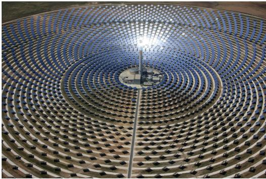
(a) Tower at the center of heliostat field
