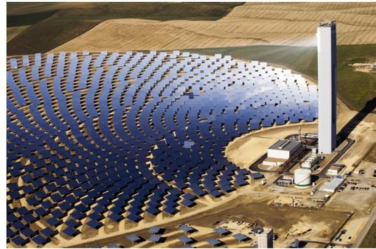
(b) Tower at the edge of heliostat field
