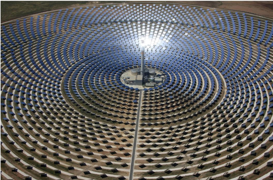
Figure 1: Image of the Gemasolar in Spain consisting of 2650 heliostats [11].
