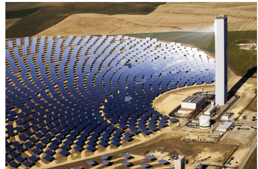
Solar tower power plant PS10 in Spain.
